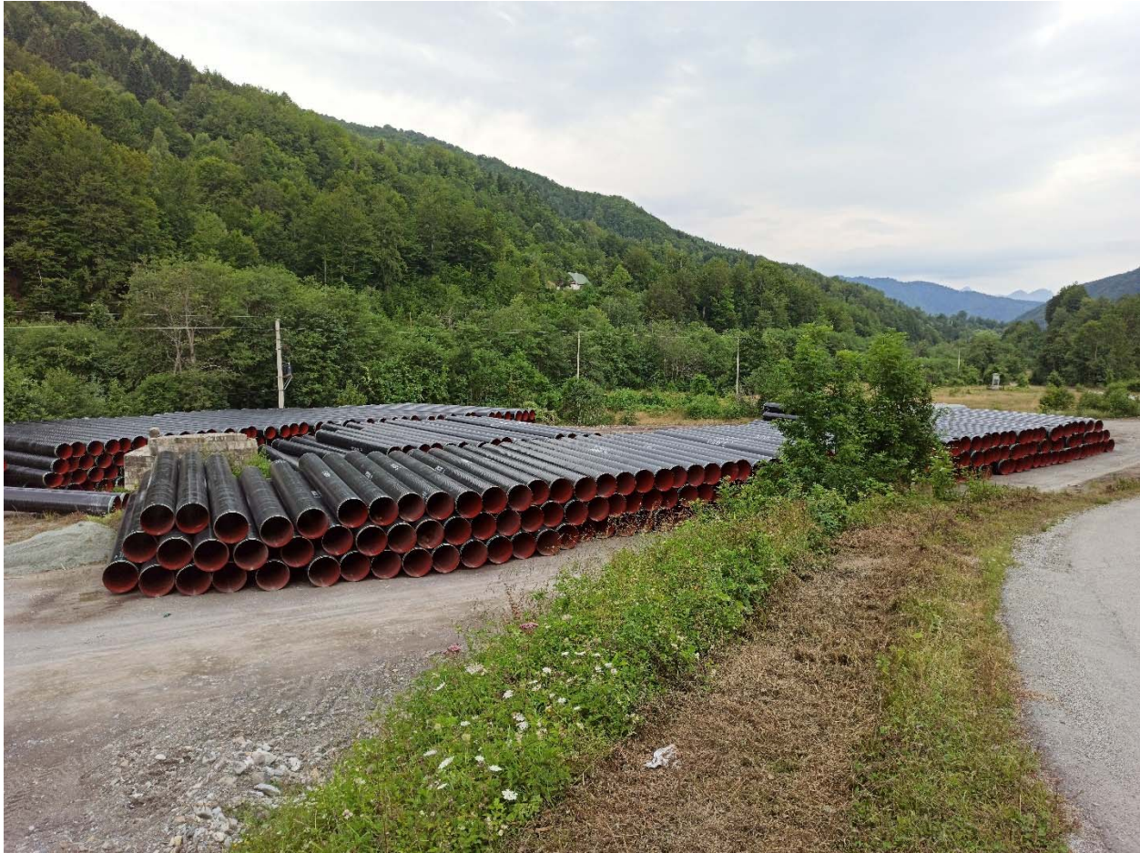
Water pipes on stock at Bara Kraljska construction site
